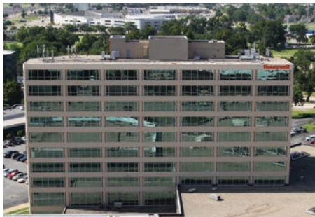
Honeywell UOP Callidus headquarters - Tulsa, Oklahoma. USA
